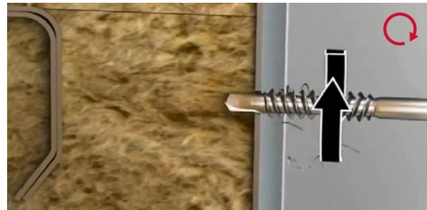
Drilling outer sheet (**clockwise – right**)
